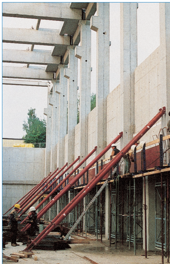
Type BKS in use in prefab construction work
