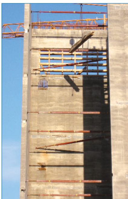
Type BKS in use in sliding shuttering work
