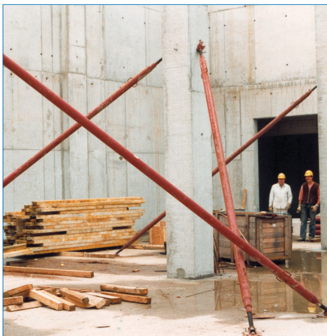
Type S in use in prefab construction work
