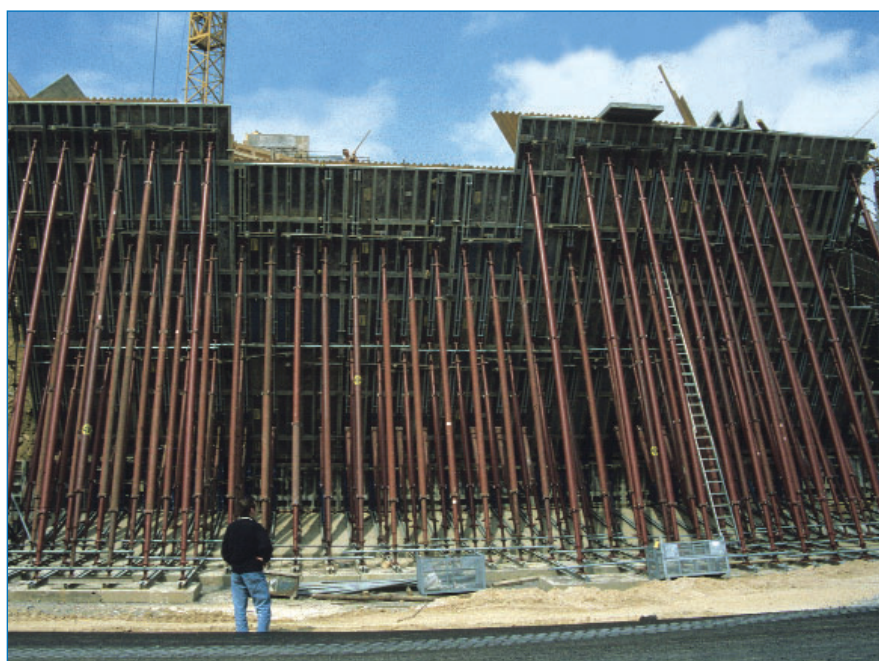
Type BKS for formwork construction: abutment of bridge construction
